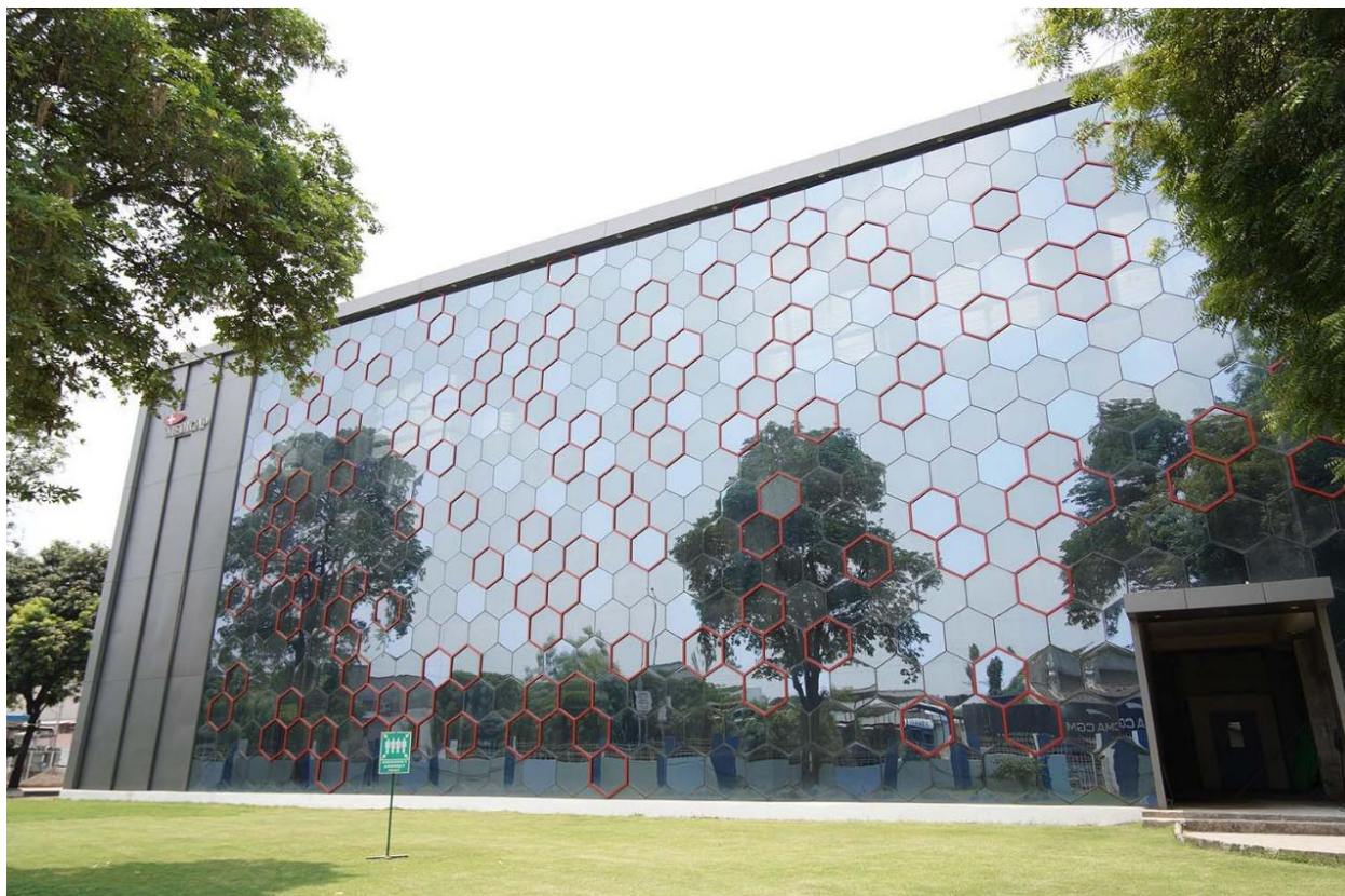
Above: E-73, GIDC, Savli, Vadodara – Manufacturing Unit
